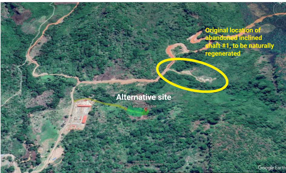
Measure 4.1: Relocation of exit of inclined shaft #1 to alternative site to avoid area of chimpanzee activity.
