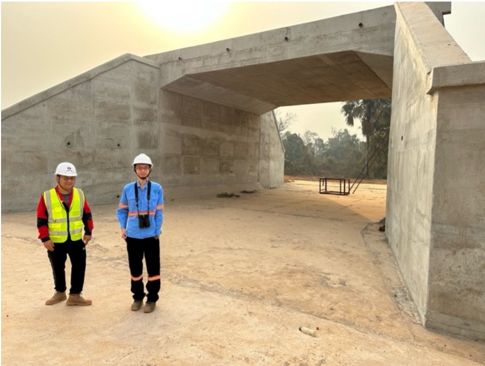
Measure 1.8: An example of a culvert under the railway which also functions as an animal passage.
