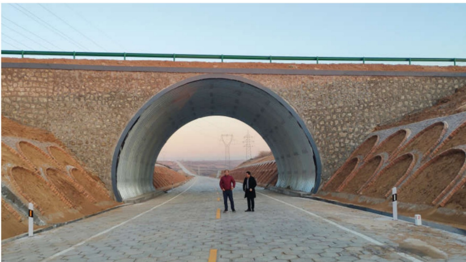
Measure 1.8: A corrugated bridge serving as an eco-flyover (example from other projects).
